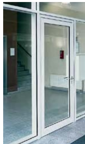
Garage and fire doors
