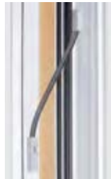
transfer of the signal cable from frame to casement
