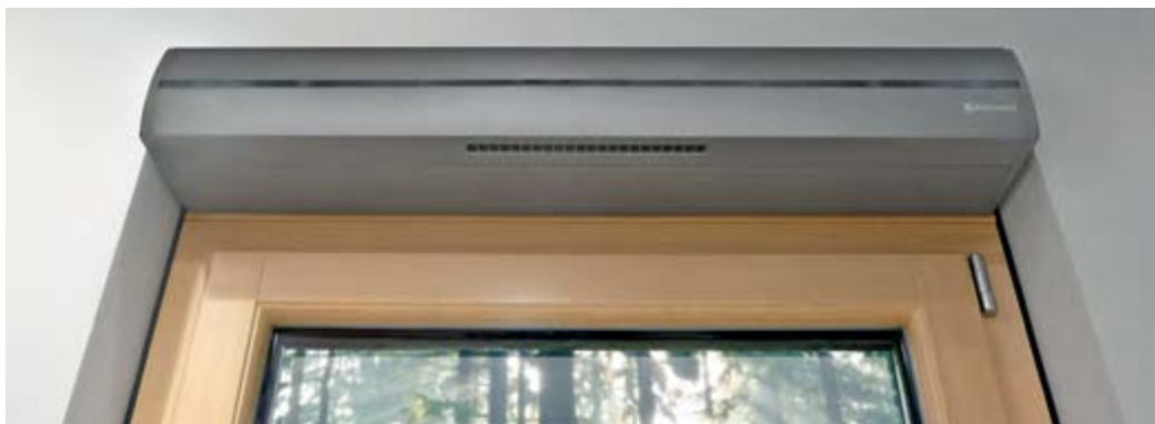
MIKrovent system installed above the window.
