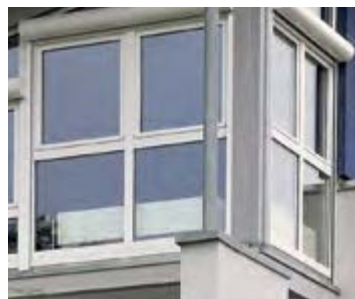
built-on roller shutter with a RONDO box
